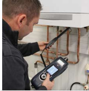
Measuring of ambient CO
